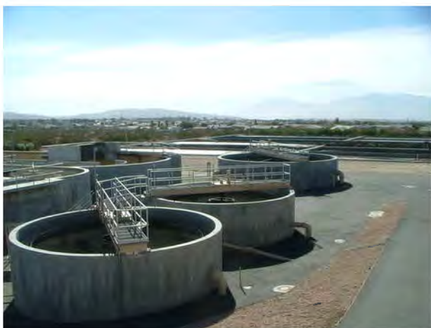
Oxidation Ditch Final Clarifiers
