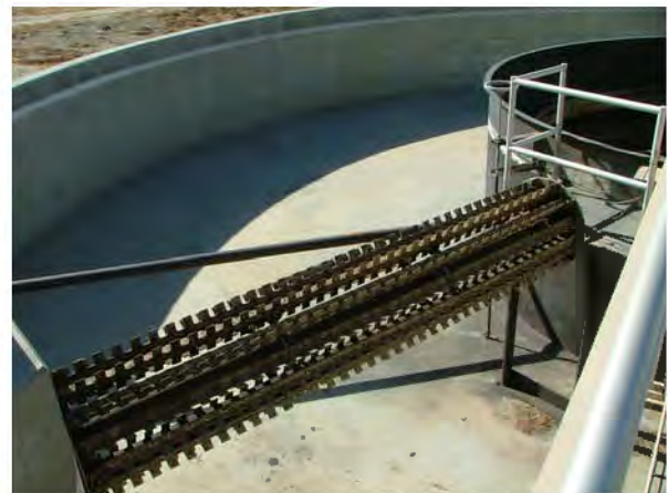
Oxidation Ditch Brush Aerator
