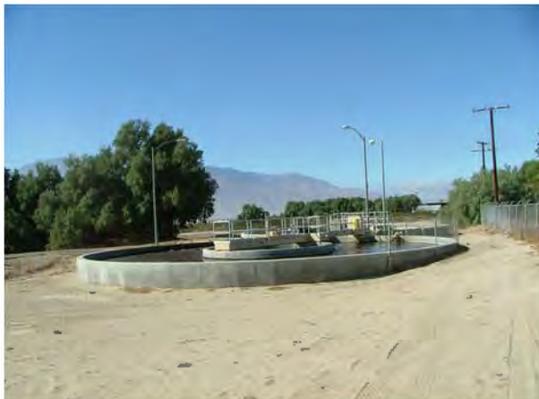
Oxidation Ditch and Clarifier
