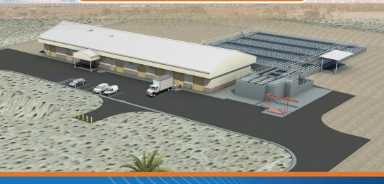
Funded primarily by grants and low-interest loans, the Regional Water Reclamation Facility will treat an additional 1.5 million gallons of wastewater per day. The expanded capacity will allow more homes currently using a septic tank system to connect. The facility will also support the addition of tertiary treatment in the future, which would provide recycled water to enhance water conservation efforts.
